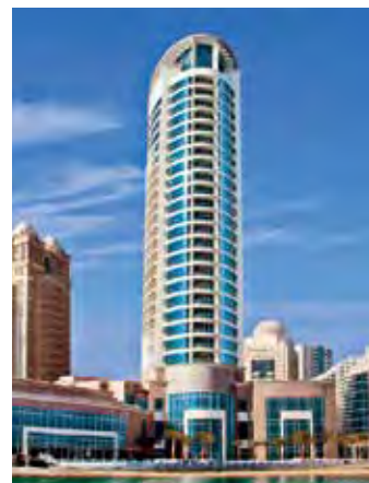
HILTON HOTEL DOHA, QATAR
