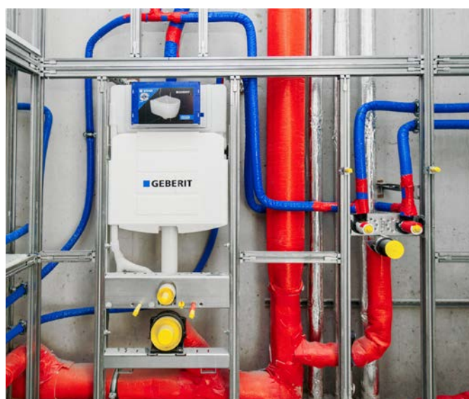
↑ GIS, introduced in 1993, is Geberit's answer to creating sanitary prewalls in drywall construction. It is particularly suitable for the prefabrication of complete sanitary walls, which speeds up installation on the construction site.
