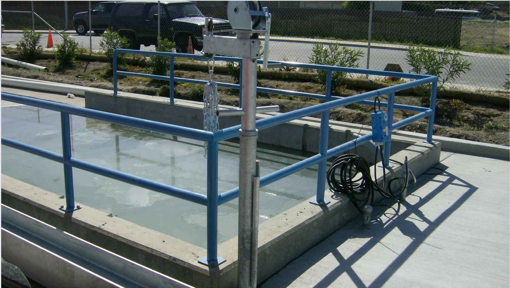
YARD WATER IS COLLECTED BY "BOAT RAMP" AND PUMPED INTO PLASTIC STORAGE TANKS FOR RE-USE
