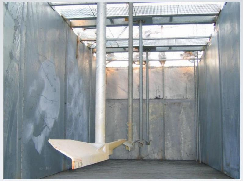
EXPANDABLE GALVANIZED ABOVE GROUND SLURRY TANKS 3 HP MOTOR AGITATORS KEEP SLURRY IN SUSPENSION. MOTORS OPERATE 5 MINUTES ON AND 10 MINUTES OFF
