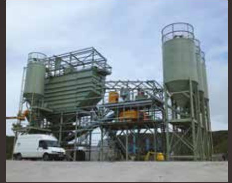
Readymix concrete, Aggregate Industries - Bardon Glasgow, Scotland
