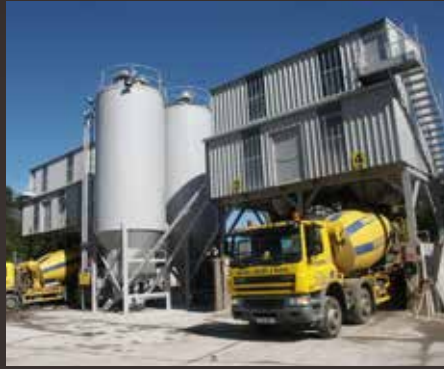
Readymix concrete CES Quarry Products Ltd Saintfield, Northern Ireland
