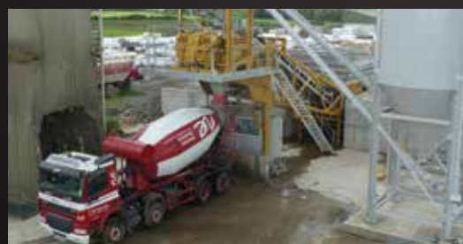
Readymix concrete Northern Ireland
