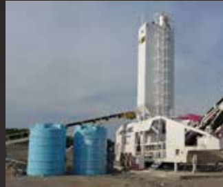
Dam building Mexico
