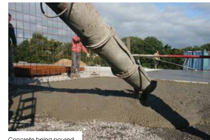
Concrete being poured
