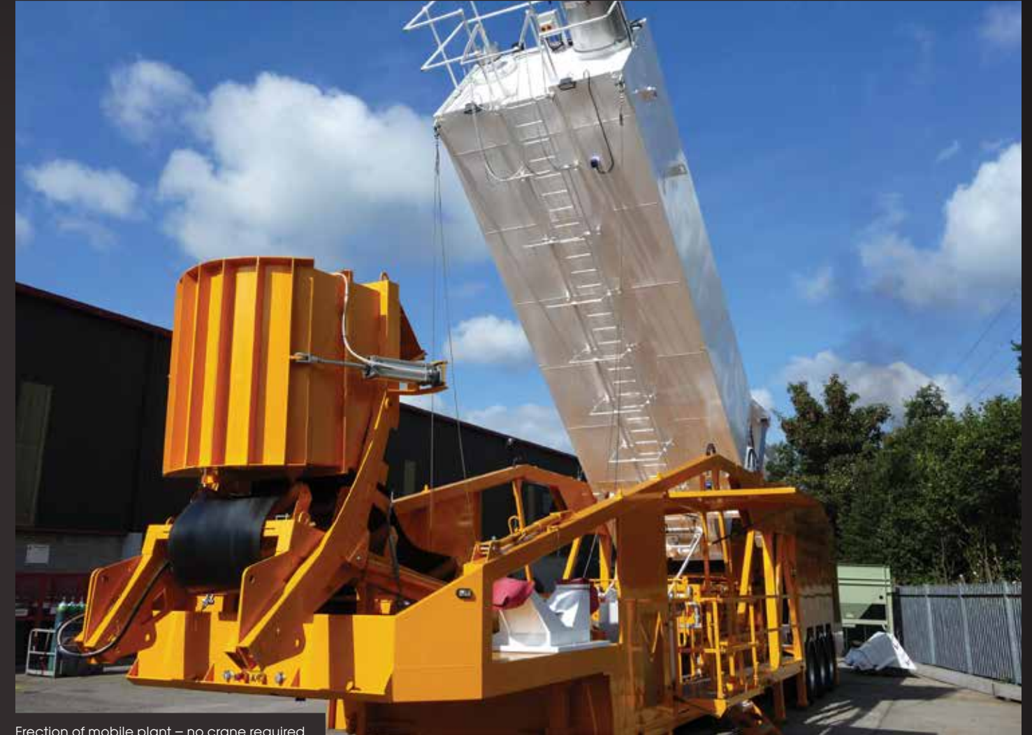
Erection of mobile plant – no crane required
