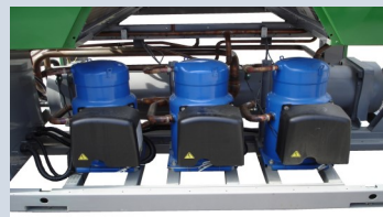
Multiple Scroll Compressors
