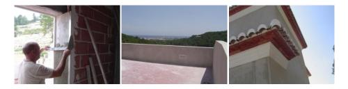
8. <u>ROOFING:</u> Will be placed over the last floor or ceiling, small walls of ceramic blocks will be constructed to form the pitches, this will in turn be waterproofed with
