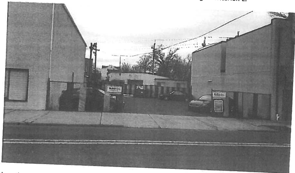
Location: 20 Union Avenue (Block 78, Lot 5 including 6) Description: Parcels are utilized as off-street parking for B&C Auto Service across Union Avenue, a non-conforming use detrimental to achieving the intended goal of the B-3 District.
