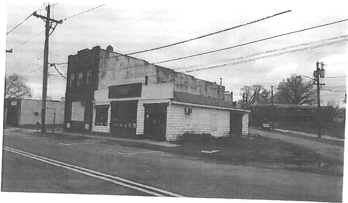
Location: 25 West Erie Avenue (Block 78, Lot 18 including 19), occupied by Pool & Spa In Town. Description: One-story commercial building on Lot 18 and a ruinous asphalt parking lot on Lot 19 located. The dilapidated building and site conditions relate to Criterion A.
