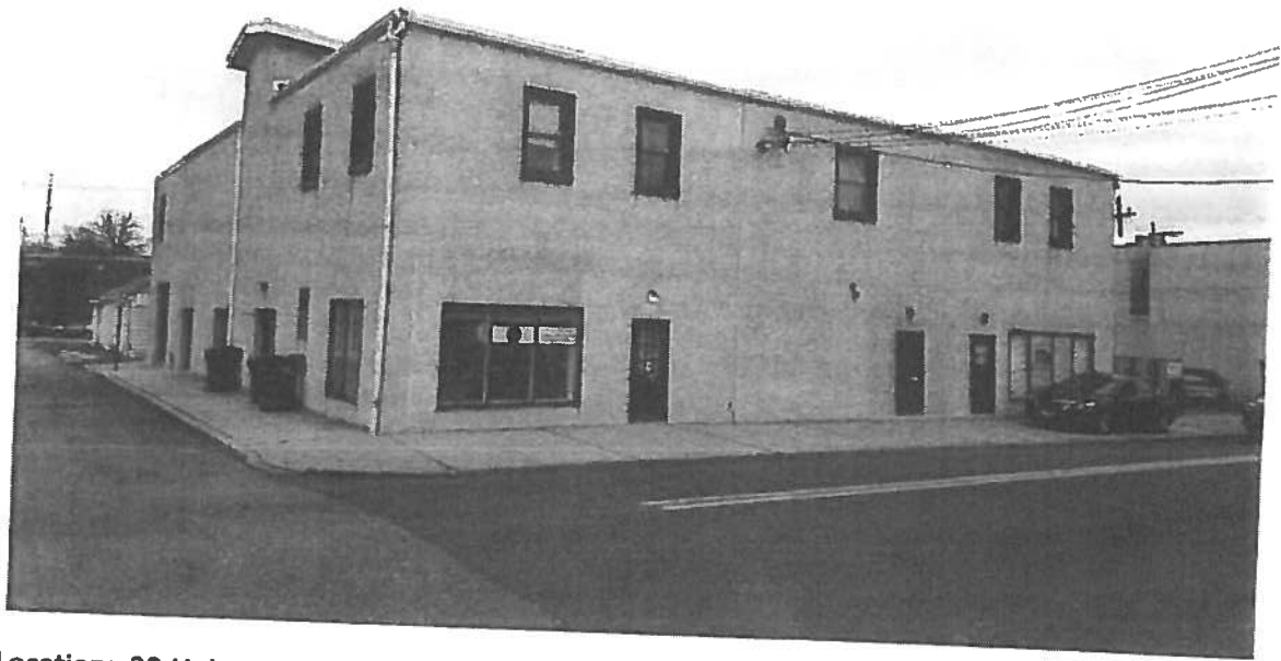
Location: 22 Union Avenue (Block 78, Lot 7), occupied by JCS Realty and Church Alive NJ. Description: Two-story industrial building with tenants utilizing first floor office space. Signs displayed in second story windows indicating vacancies, relating to Criterion E.
