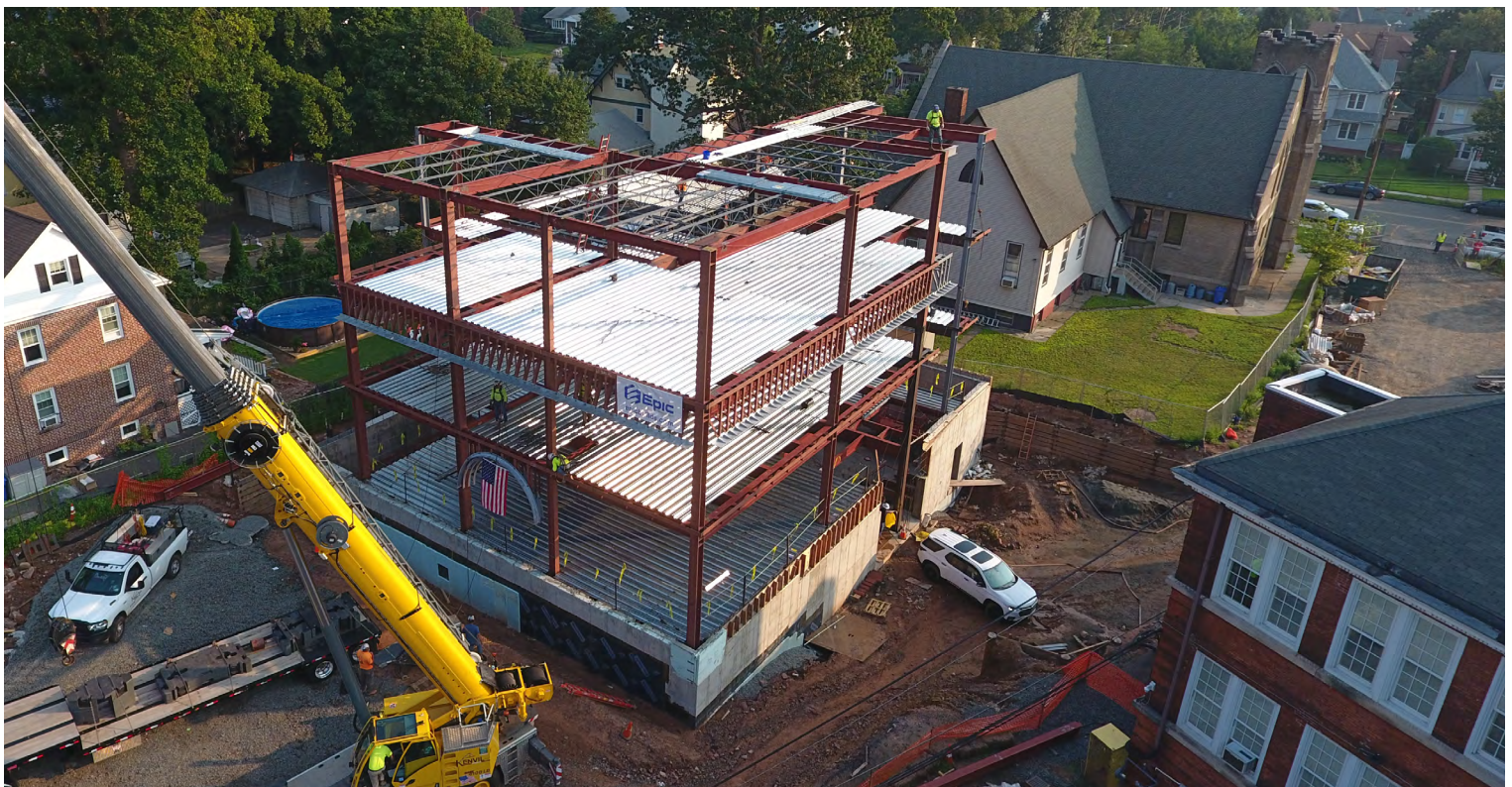
Recent drone photos of the new RPD Headquarters
