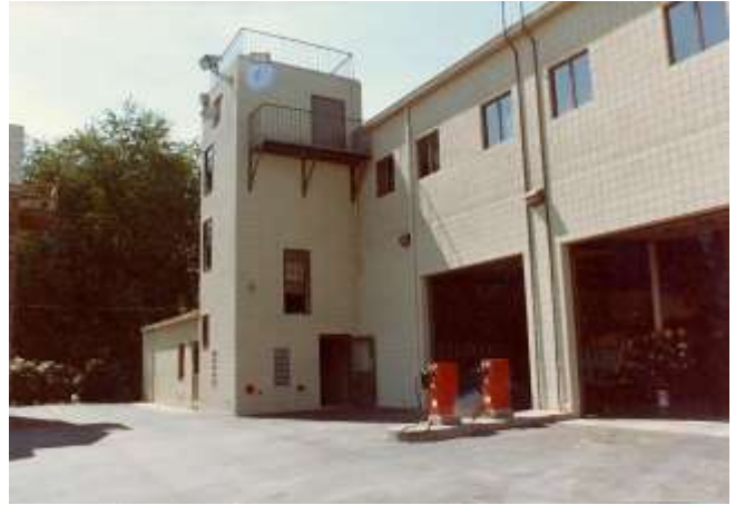
Rear of STMFD station.
