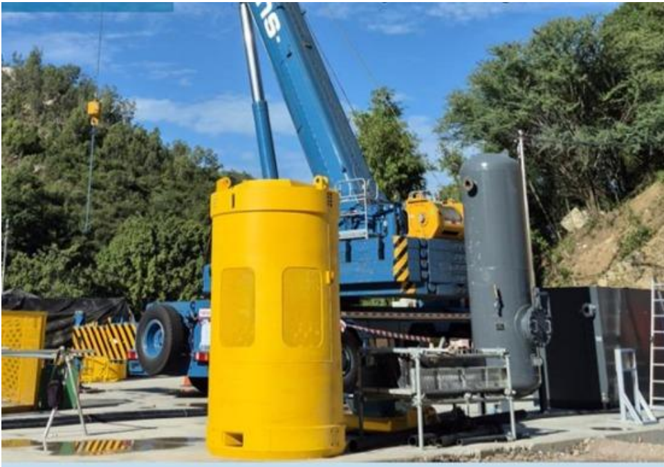
Figure 15. Shaft Sink Construction (Equipment Kibble)
