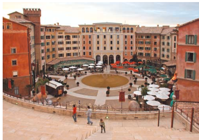
Foto: Siemens Building Technologies
