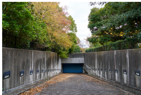
Underground Parking Lot (Within Aomi Minami Port Park) Started to use in April 1997, this parking facility with an area of 7,603.75 square meters accommodates 216 vehicles.
