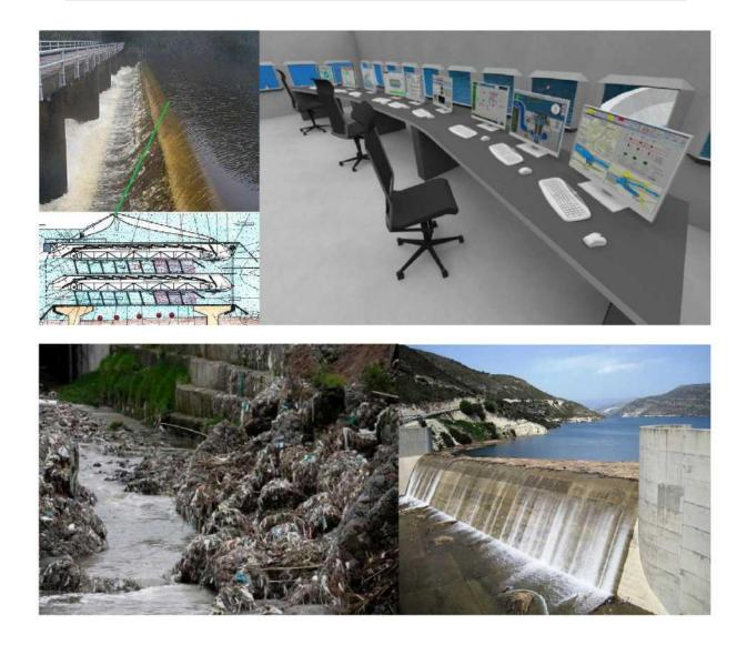
The management of all processes of the described operation of the cascading hydroelectric power plant is from the monitoring room, from where everything is managed including automatic cleansing of the surface waste from the river, which deposits on an anchored barge and is then easily taken away
