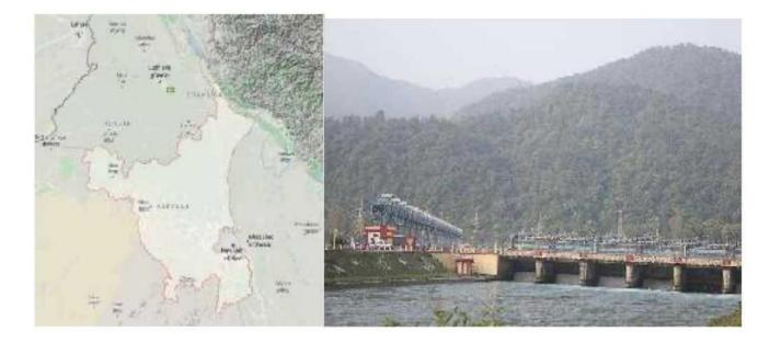
From the mentioned lock until the New Delhi, the river drop of the Yamuna River can be utilized with an altitude difference of 250 meters, that is sufficient fall of the river bed to build 100 CHPP with an average cascade height of 2.5 m 50% of the Yamuna River is already used in the irrigation process, while the other 50% would be used for the construction of the CHPP
