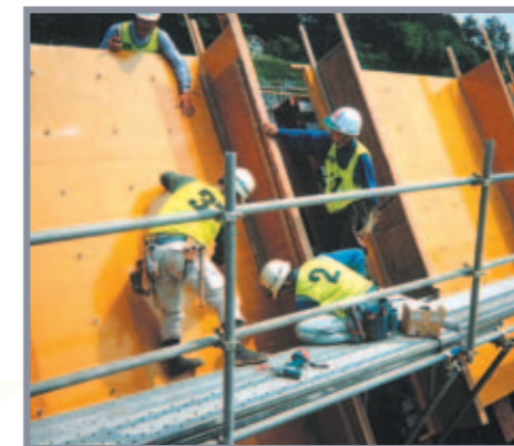
SAMM sheet placing work (placing work on compressed diagonal material)
