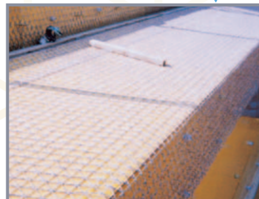
Placed SAMM sheet (Wooden formwork)
