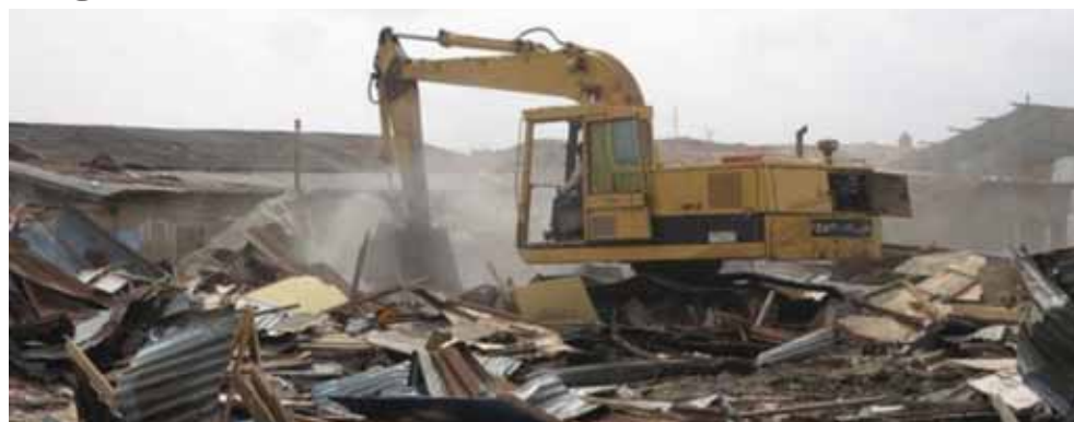
A view of Badia-east Demolition Exercise
