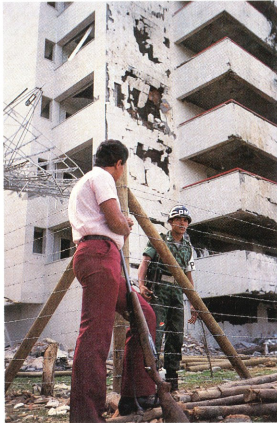
"Don" Pablo Escobar's bombed-out apartment building
