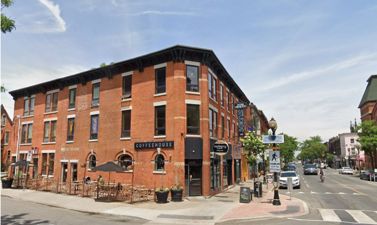
193 James Street North, Hamilton, Ontario
