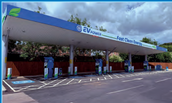
EV Charging Hub
