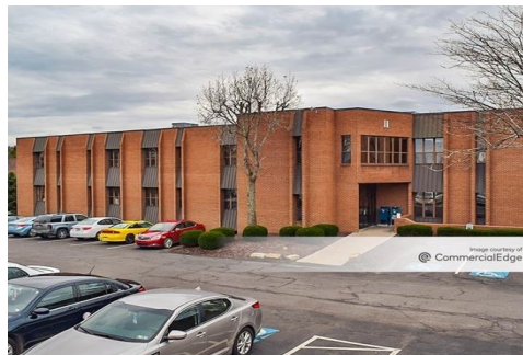
Front of building (Perry Hwy side)
