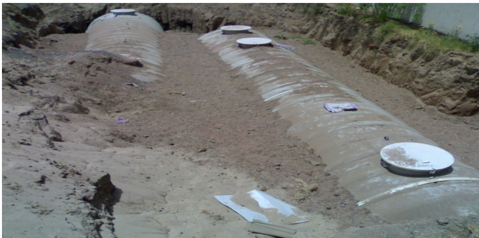
C) Filling By pebbles & Soil up to the manhole level:
