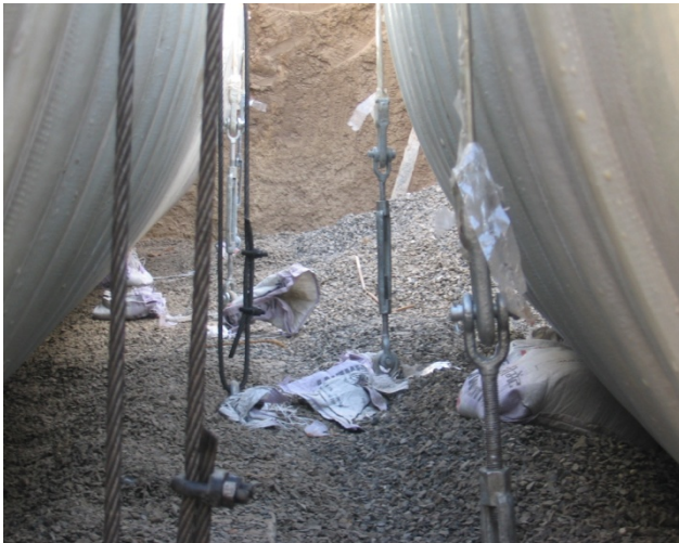
C) Filling By pebbles & Soil up to the manhole level:
