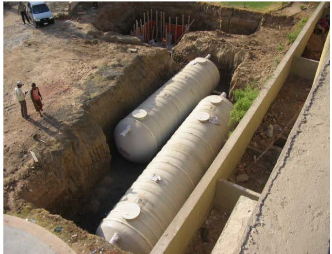
C) Filling By pebbles & Soil up to the manhole level:
