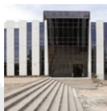
MADRID GLOBOMEDIA PROJECT BY BNB PROJECT
