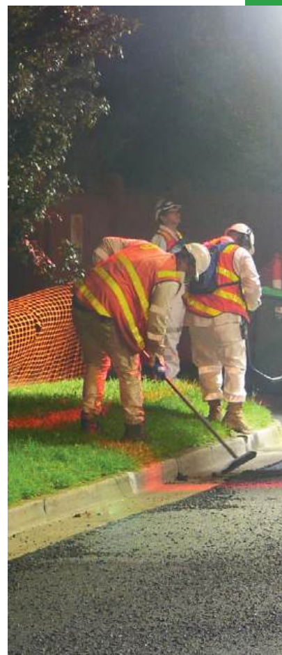
New road project in Bentleigh, Victoria.
