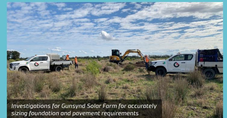
Investigations for Gunsynd Solar Farm for accurately sizing foundation and pavement requirements
