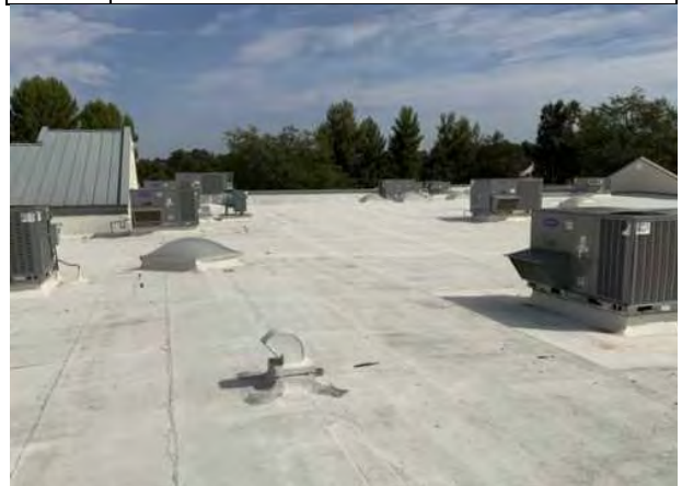
#28: MODIFIED BITUMEN ROOFING
