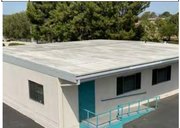
#30: SINGLE-PLYTPO/PVC ROOF MEMBRANE
