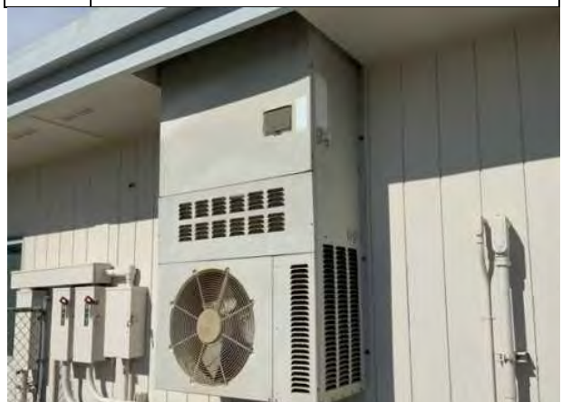
#42: WALL-MOUNTED PACKAGED UNIT
