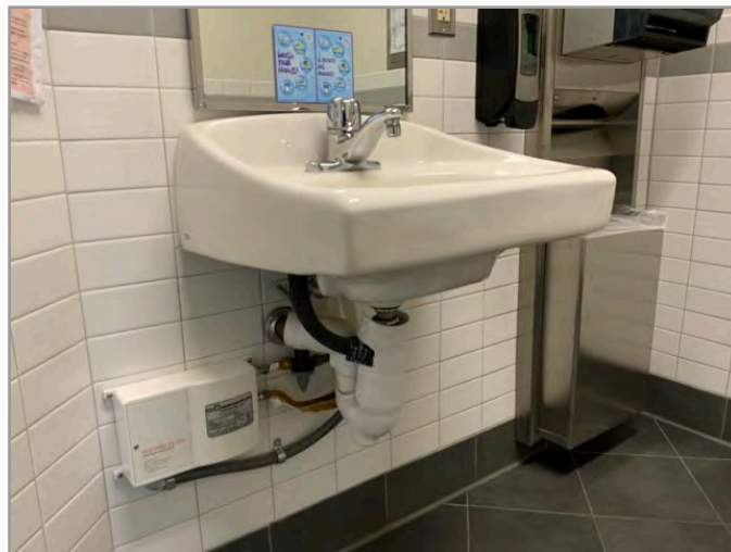
Sink, faucet handles and under counter clearances
