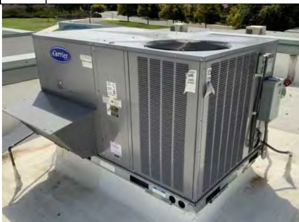
#41: ROOFTOP PACKAGED UNIT (RTU)
