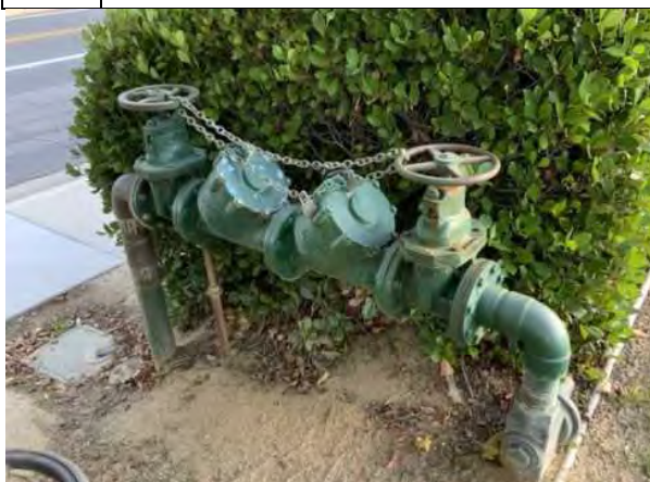
#59: DOMESTIC WATER BACKFLOW PREVENTER
