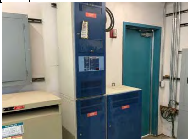
#47: EMERGENCY BACKUP INVERTER FOR LED LIGHTING
