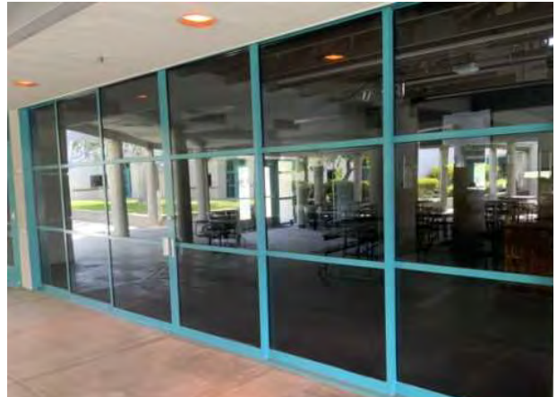
#20: EXTERIOR GLAZED LARGE SLIDING DOOR
