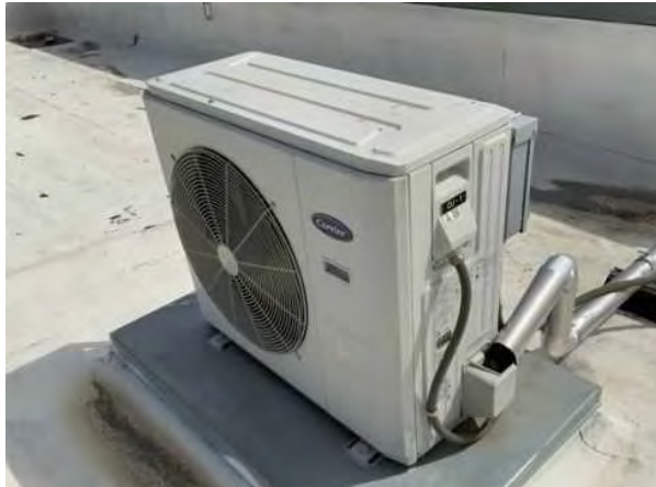
#43: DUCTLESS SPLIT SYSTEM COMPONENT
