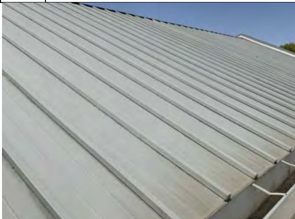
#29: METAL ROOFING WITH GUTTERS
