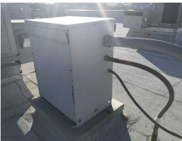
35 - SECONDARY TRANSFORMER
