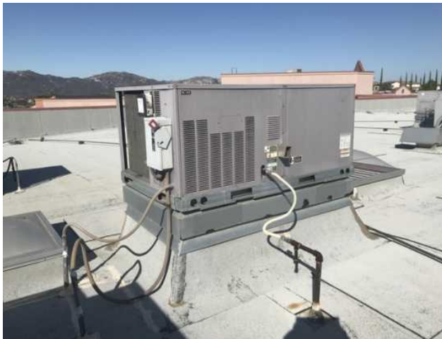
27 - PACKAGED UNIT, RTU
