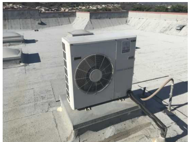
30 - SPLIT SYSTEM DUCTLESS
