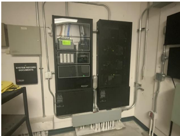
27 FIRE ALARM CONTROL PANEL
