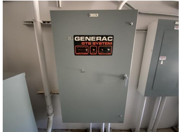
26 AUTOMATIC TRANSFER SWITCH
