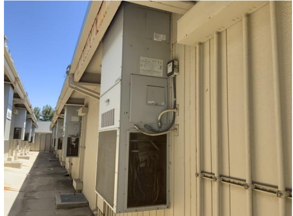
22 WALL-MOUNTED HEAT PUMP
