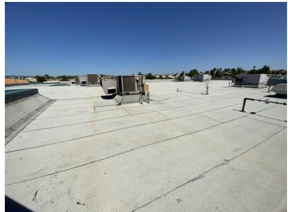
18 MODIFIED BITUMEN ROOF
