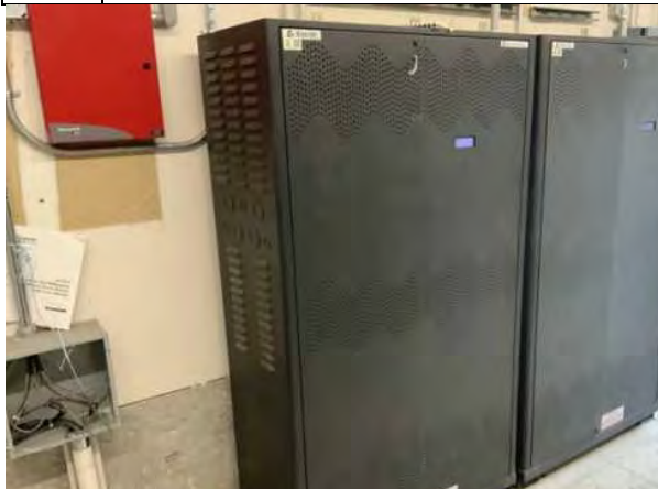
#45: BACKUP INVERTER LED LIGHTING
