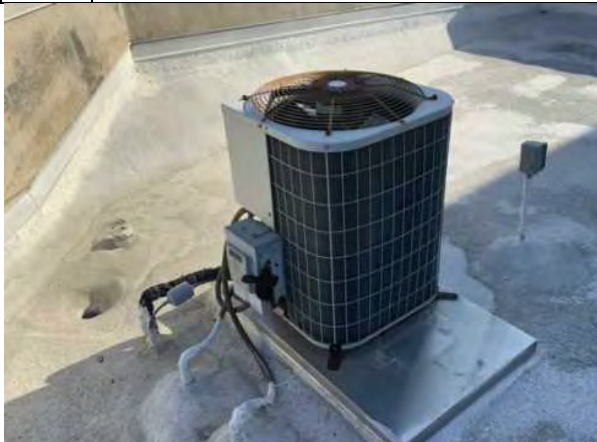
#41: EXTERIOR SPLIT SYSTEM COMPONENT
