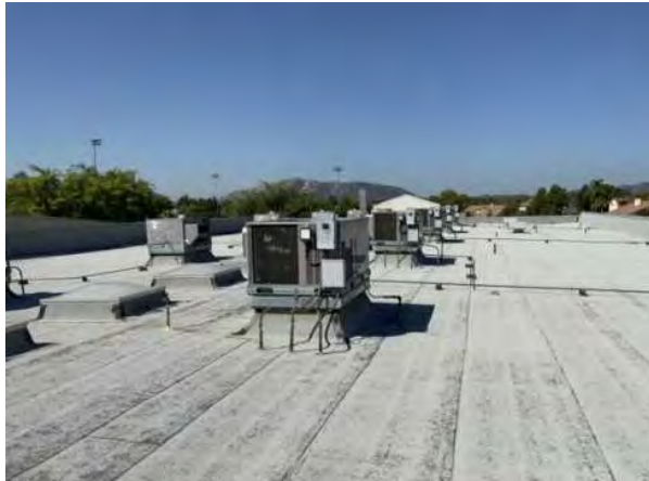
#25: MODIFIED BITUMEN ROOFING
