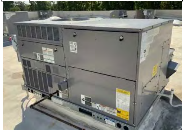
#40: ROOFTOP PACKAGED UNIT (RTU)
