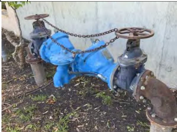
#59: DOMESTIC WATER BACKFLOW PREVENTER
