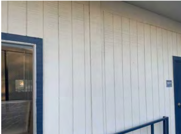
#19: EXTERIOR PLYWOOD/OSB WALLS
