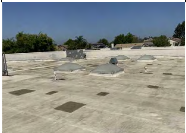
#24: MODIFIED BITUMEN ROOFING WITH FOAM
