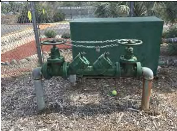
#29: DOMESTIC/WATER/BACKFLOW PREVENTER
