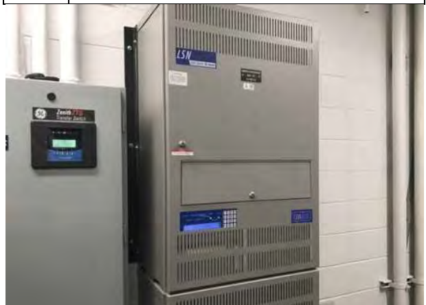
#40: UNINTERRUPTIBLE POWER SUPPLY
