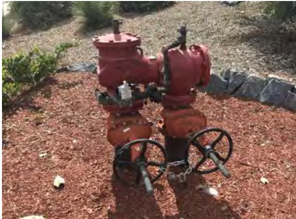
#37: FIRE WATER BACKFLOW PREVENTER
