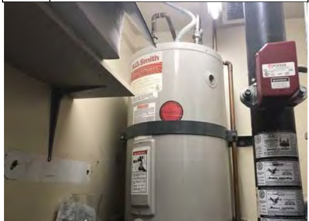
#28: ELECTRIC WATER HEATER
