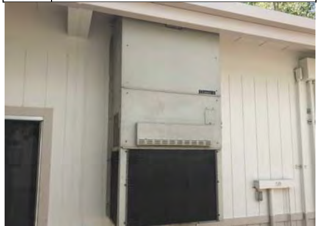
#34: WALL MOUNTED HEAT PUMP
