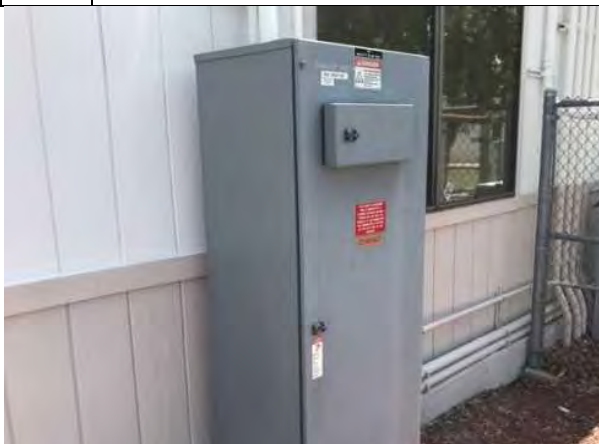
#39: AUTOMATIC TRANSFER SWITCH
