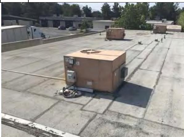
#35: ROOF TOP PACKAGED UNITS
