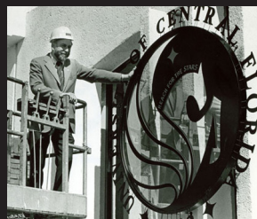
UCF President Colbourn stands in a cherry picker, with the newly installed school seal on the Administration Building (now Millican Hall).
