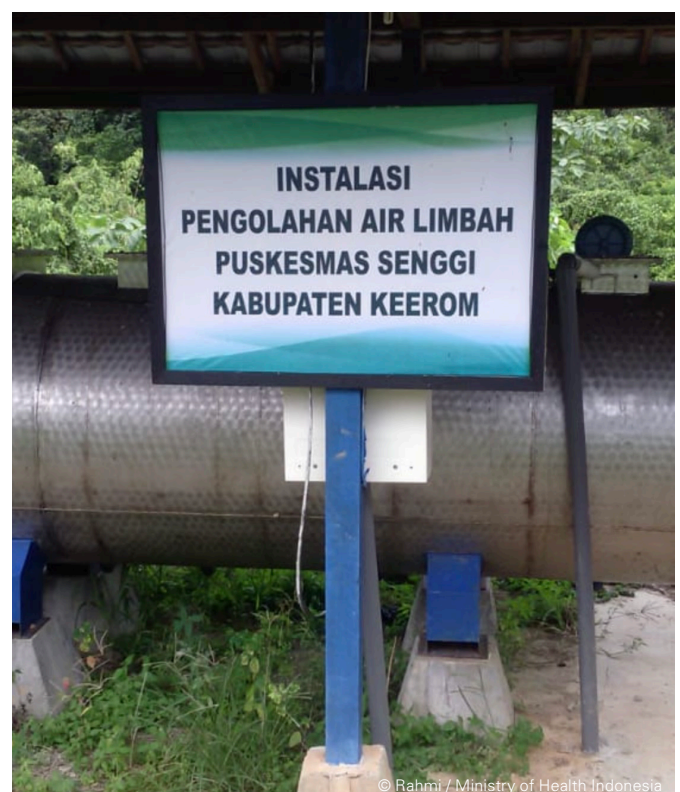
Wastewater treatment facility in Puskesmas in Keerom District, Papua
