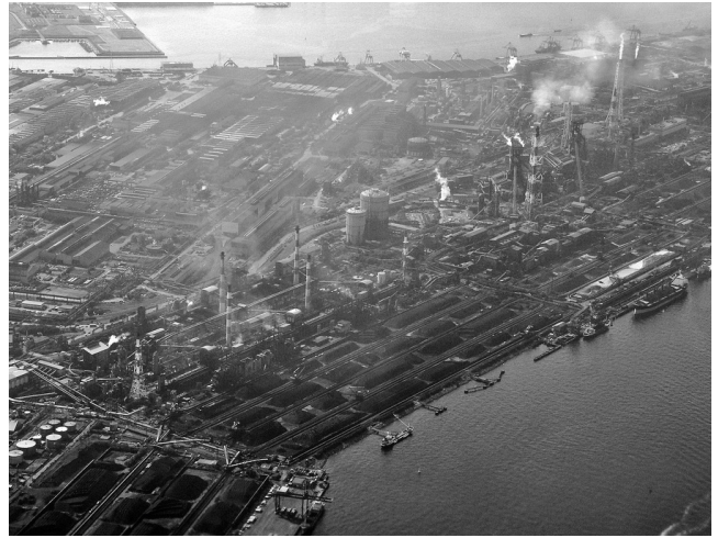
Ougijima Thermal Power Plant. Photo: Takato Marui
