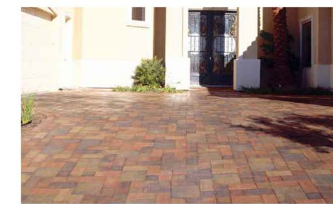
SPECIALTY PEDESTRIAN PAVING MANUF: PAVESTONE TYPE: CITYSTONE III PARKWAY COLOR: SIERRA BLEND
