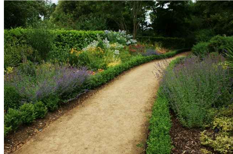
C COMPACTED DECOMPOSED GRANITE PATH
