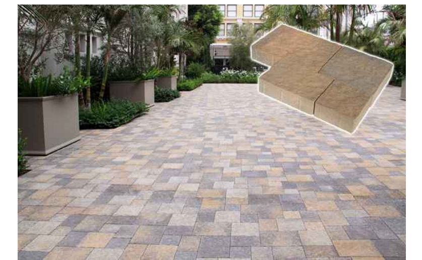
I SPECIALTY PEDESTRIAN PAVING
