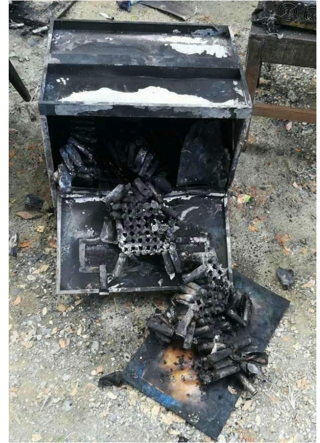
Lithium NMC battery from an off-grid solar system following a fire
