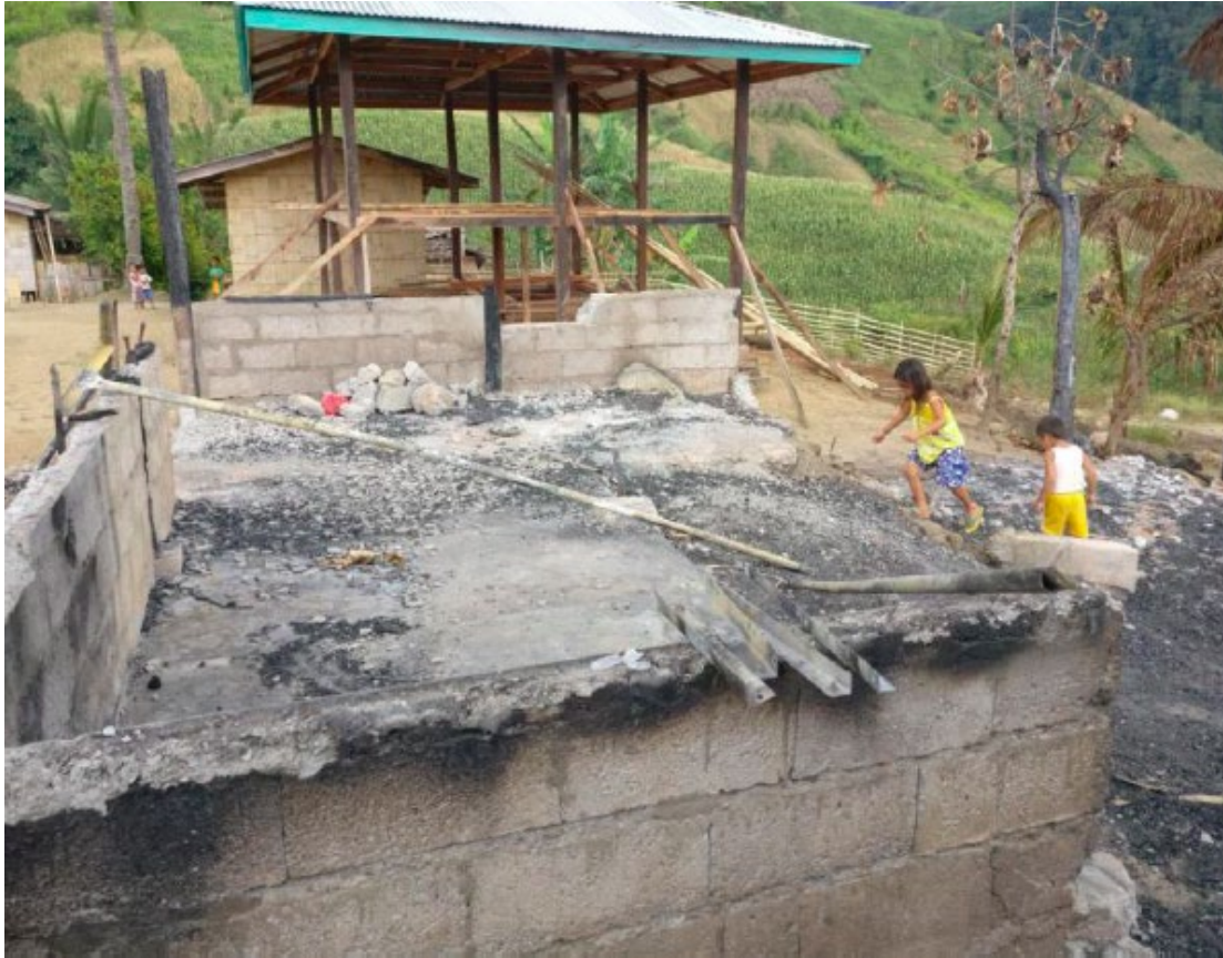
House that burned following a fire associated with an off-grid solar system that had a lithium NMC battery
