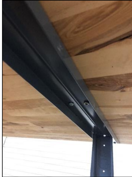
Figure 14. SWP test bench metal legs and support across screwed to the underside of the butcher block table
