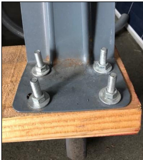
Figure 12. Metal legs bolted with hex bolts securely to the wooden base piece and approximately centered for balance and strength
