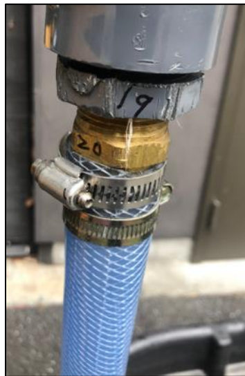
Figure 39. Adjustable non-permanent hose clamps fitting the threaded hosing to PVC adapter number 20 at the piping network's inlet- this is okay to use at the inlet to allow for any needed adjustment
