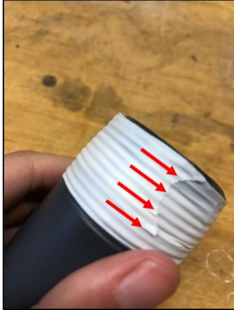
Figure 35. Plumber's tape wrapped clockwise around male-end of PVC adapter; the arrows show the direction the other piece will push against it, which should be in-line with the tape.
