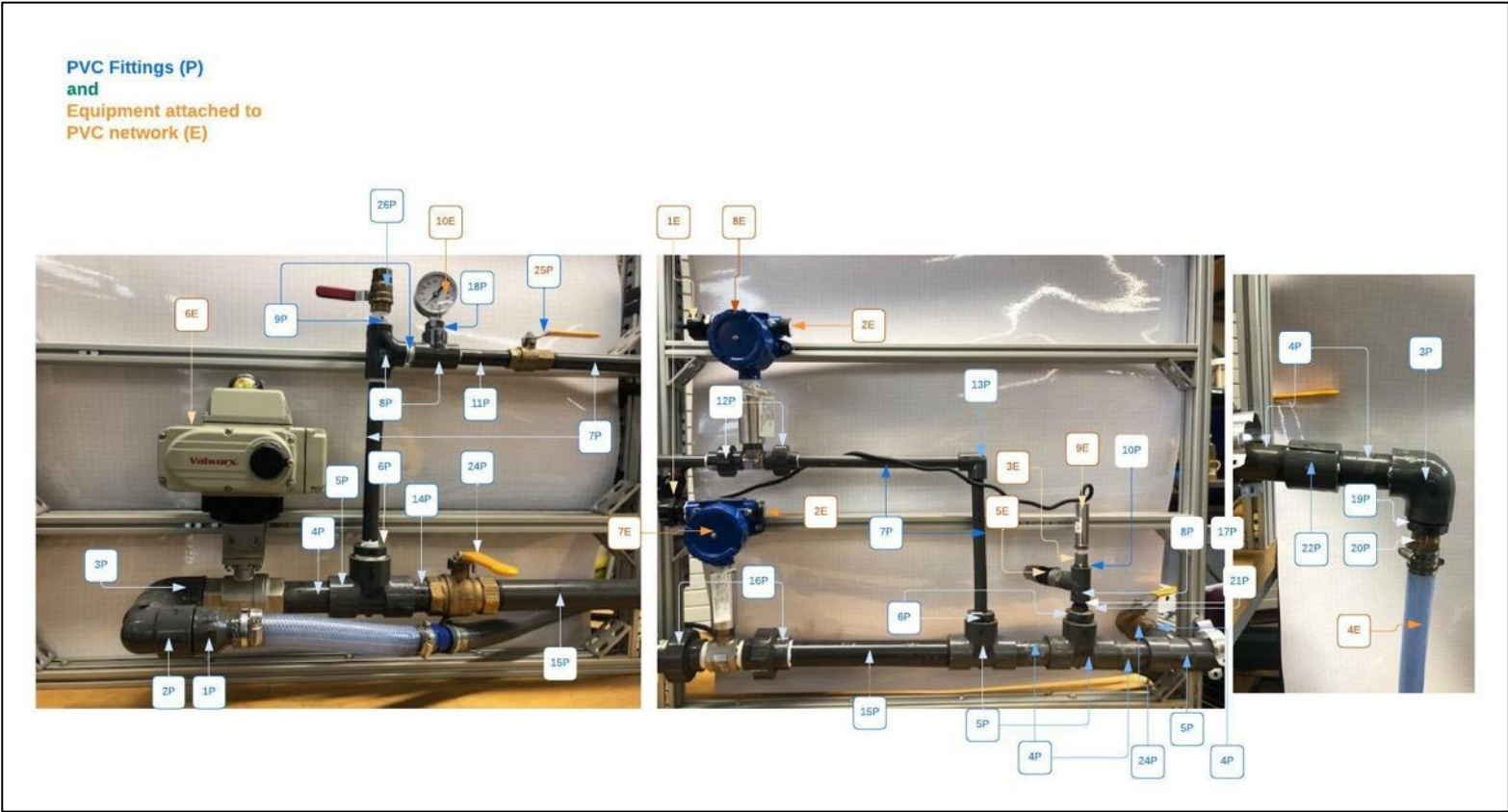
Figure 3. PVC piping network with equipment attached labeled items
