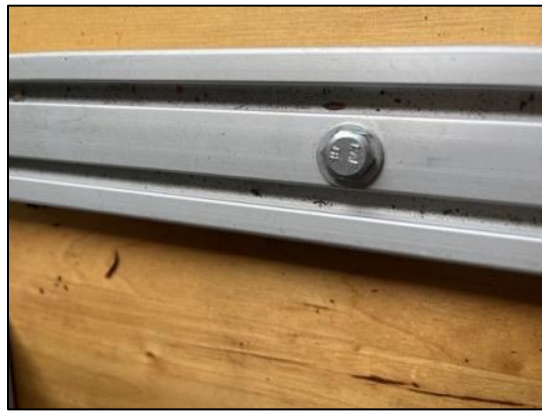
Figure 19. Hex bolt and washer driven through the t-slotted framing and into the butcher block for solid connection
