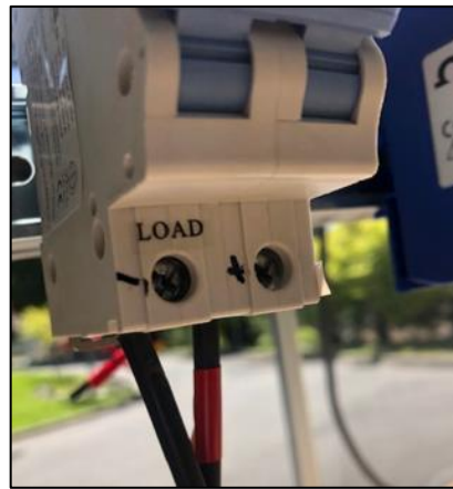
Figure 47. 16A fuse switch screw terminals
