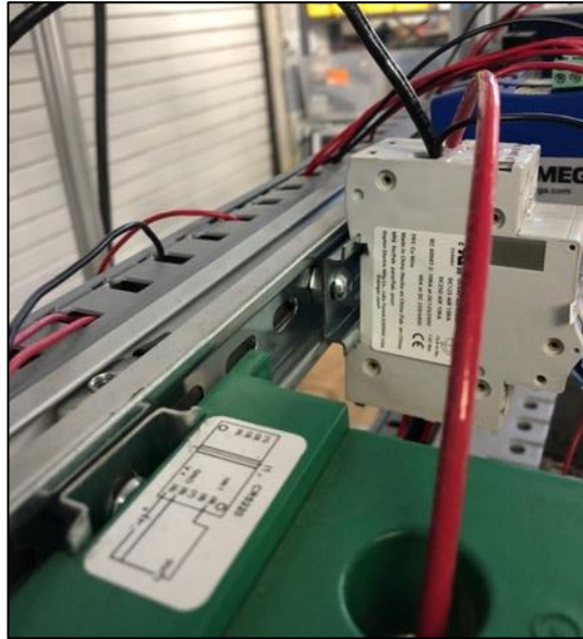
Figure 44. DAQ equipment installed using hex screws and t-nuts to the 35mm mounting track affixed to single t-slotted framing within the shielded area of the test bench
