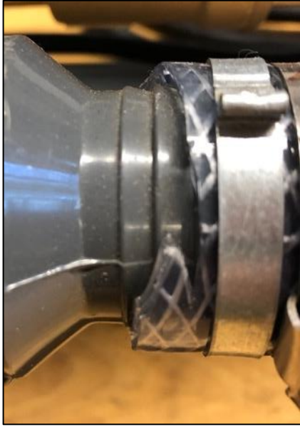
Figure 37. Hose clamp affixes threaded hose to PVC adapter on the outlet of the PVC network
