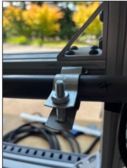
Figure 43. Low-flow PVC branch secured to t-slotted framing with 3/4" screw conduit PVC clamp
