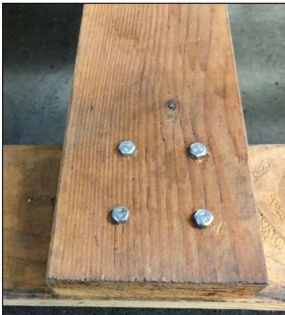
Figure 9. Wooden base bolted together to ensure durability
