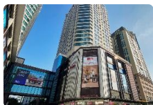
Ba Trieu Office Building
