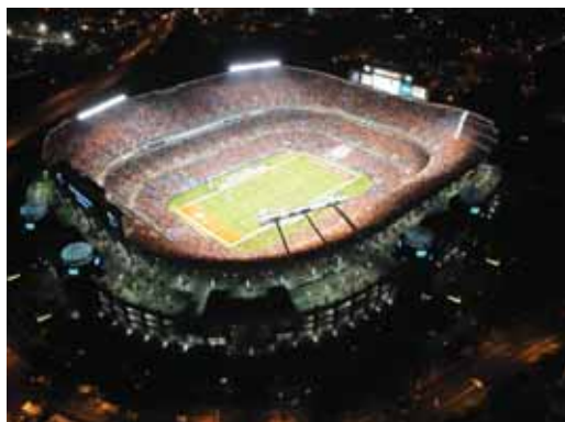
Charlotte's Bank of America Stadium
