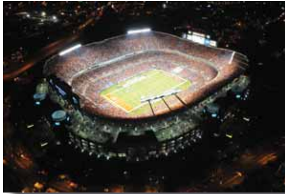
Charlotte's Bank of America Stadium
