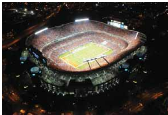
Charlotte's Bank of America Stadium
