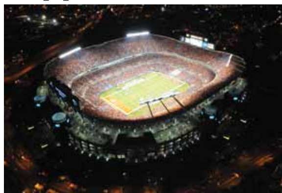
Charlotte's Bank of America Stadium
