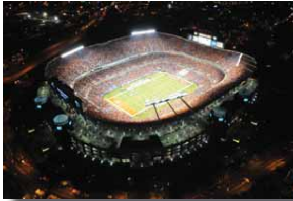
Charlotte's Bank of America Stadium
