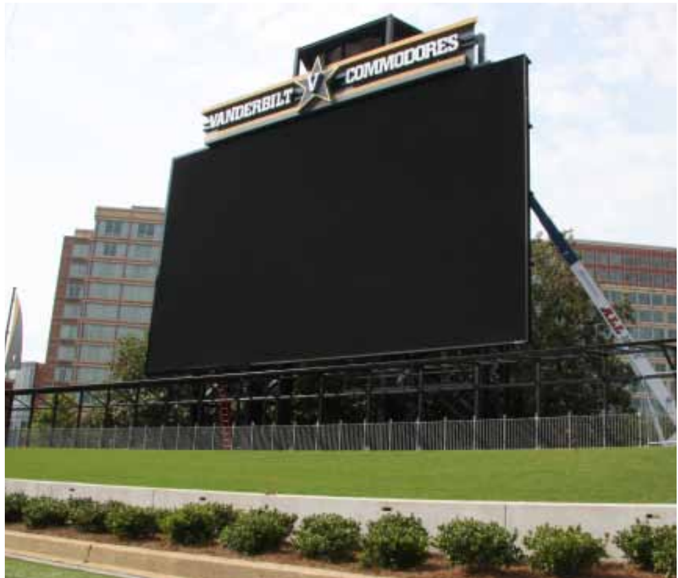
The new video board and berm in the south endzone of Vanderbilt Stadium.
