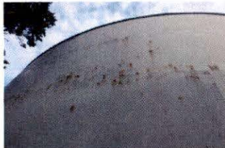
EXTERIOR COATING CORROSION
