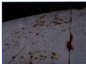
EXTERIOR COATING CORROSION
