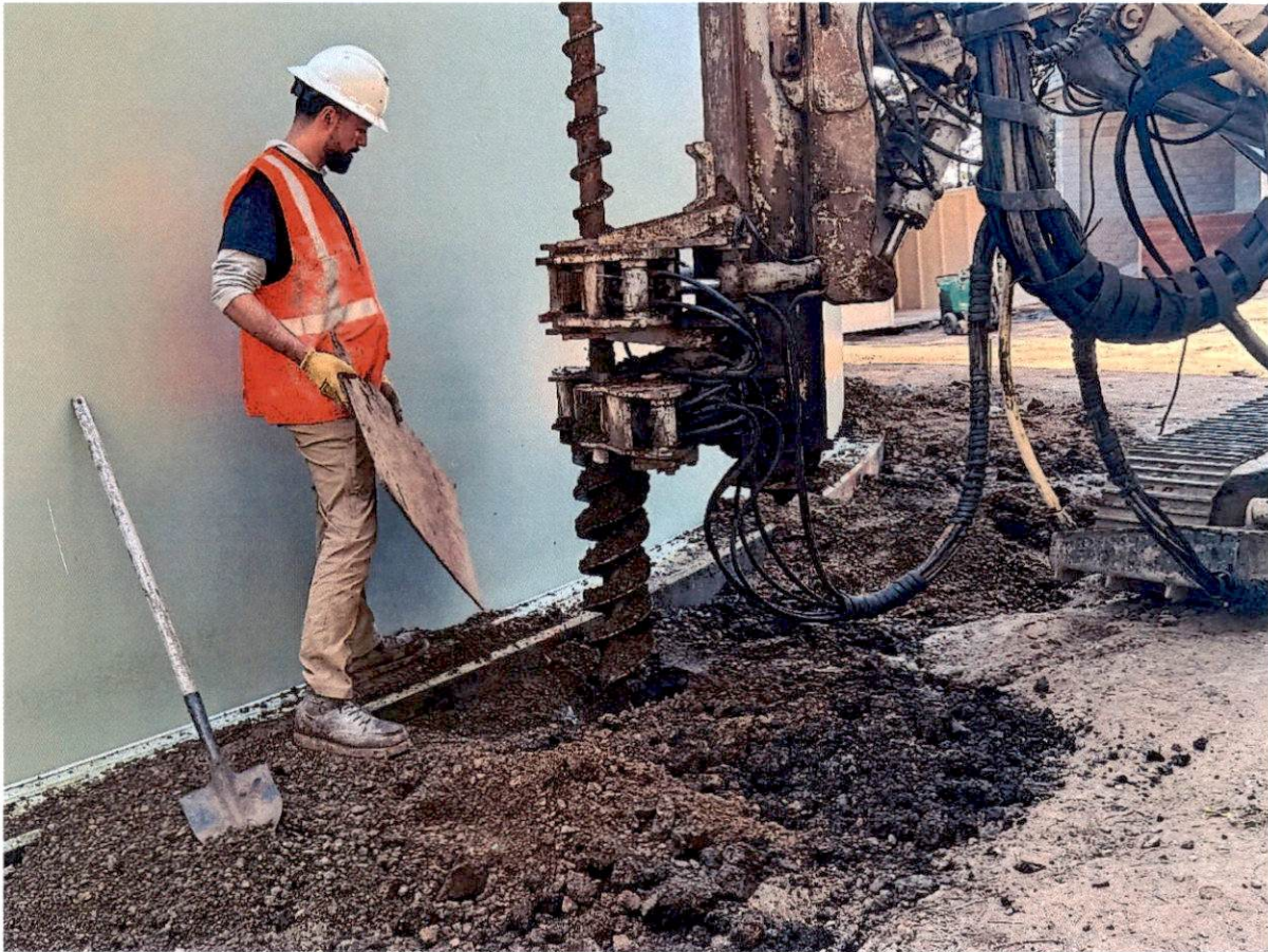
September 17, 2025 – Micropile drilling operation.
