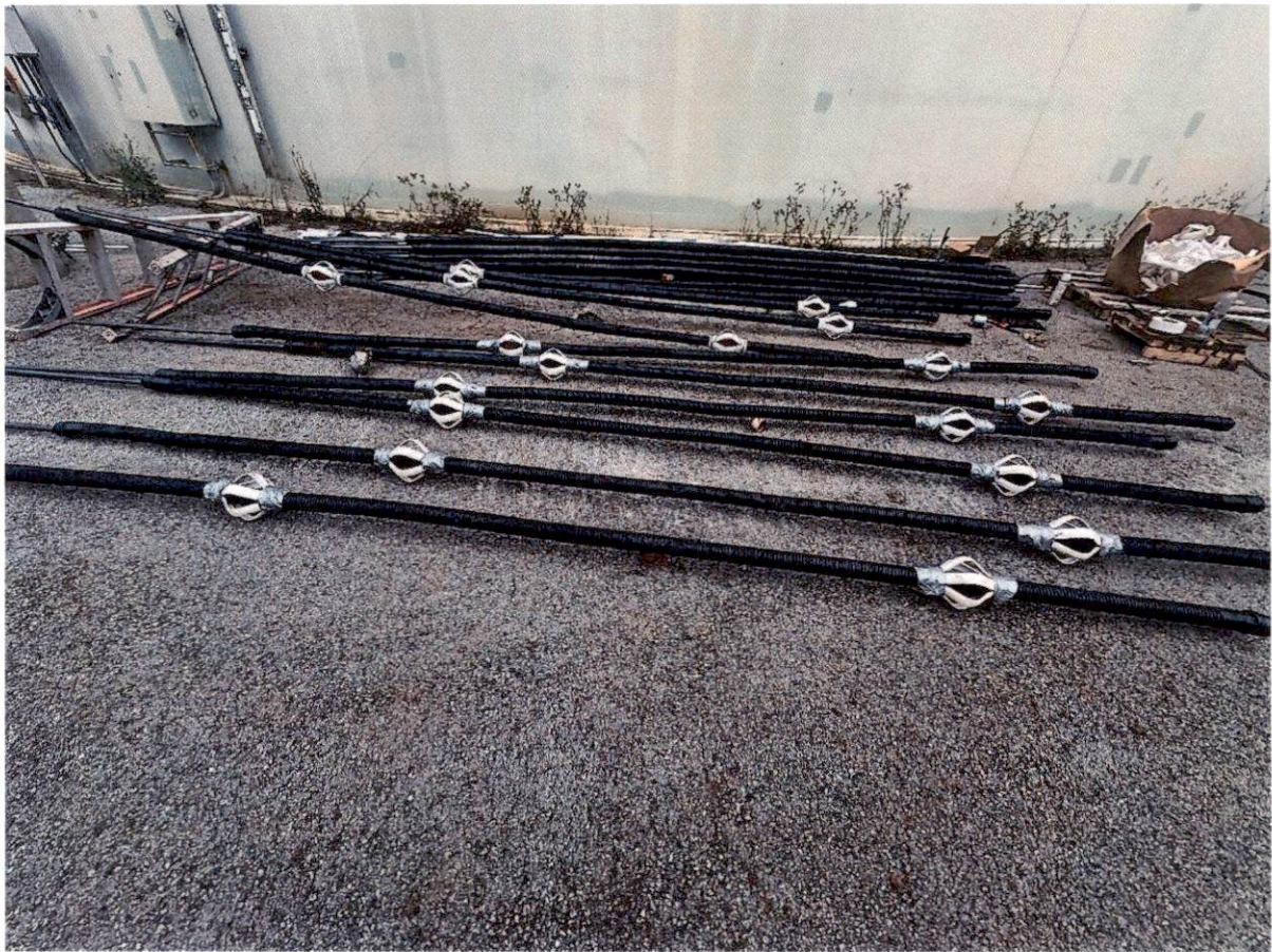
September 18, 2025 – Micropile steel bar with spacers.
