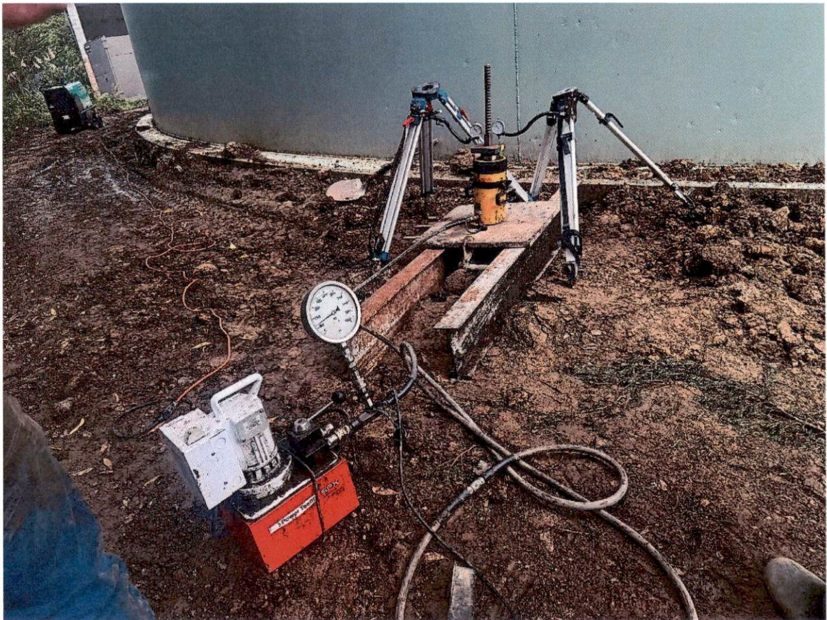
September 16, 2025 – Micropile testing operation.
