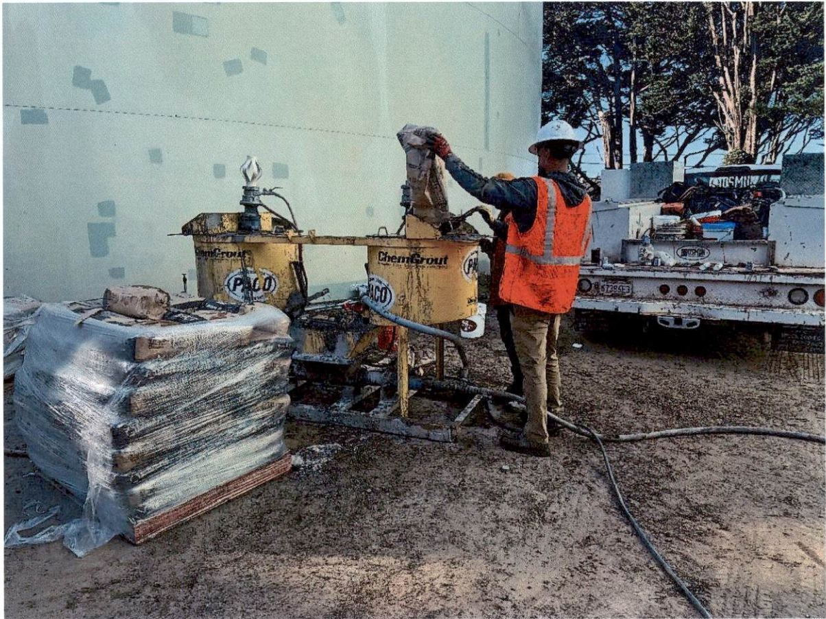
September 22, 2025 – Micropile grouting machine.
