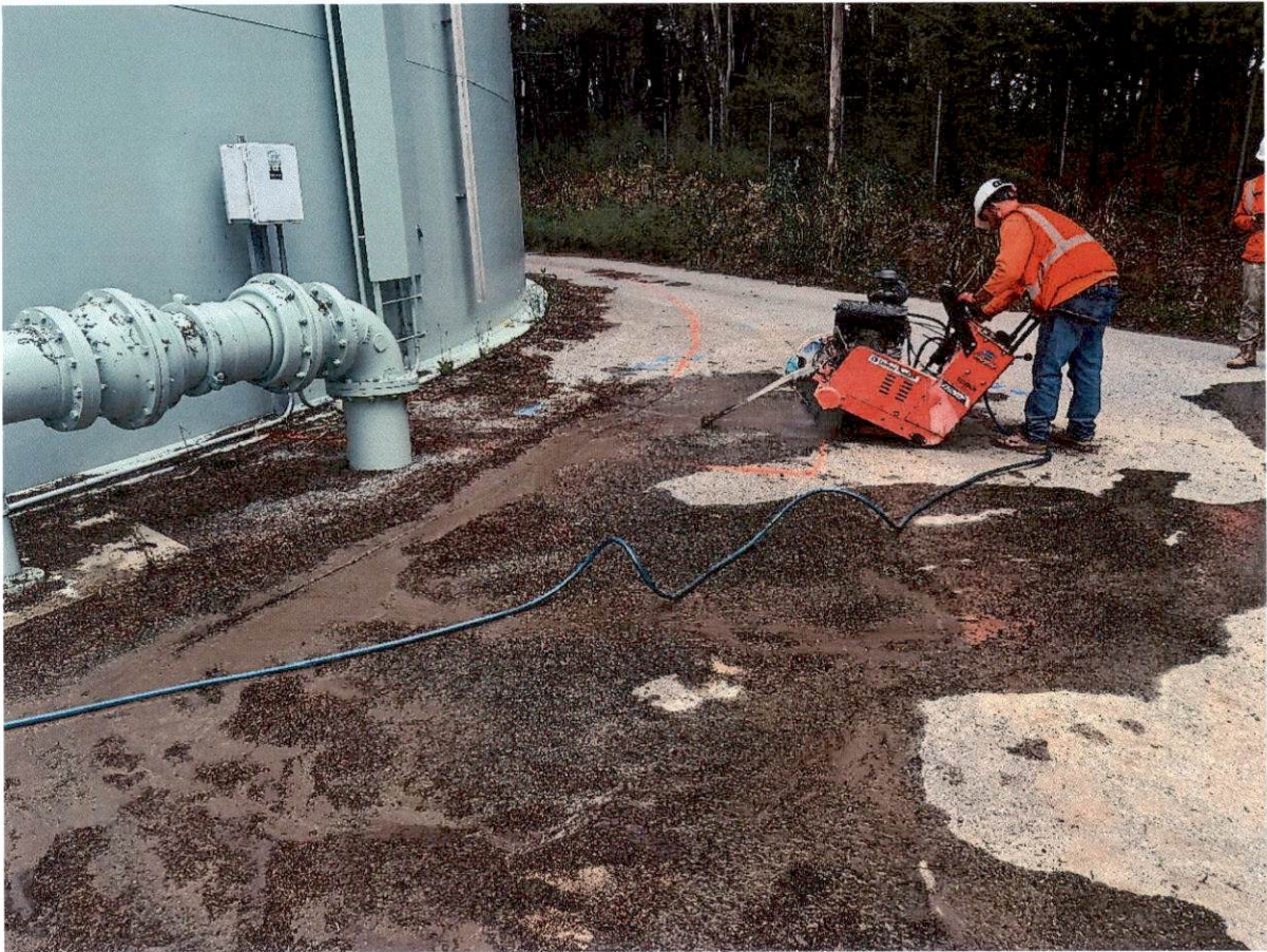
August 11, 2025 – ESM sawcutting the existing pavement to permit foundation installation.
