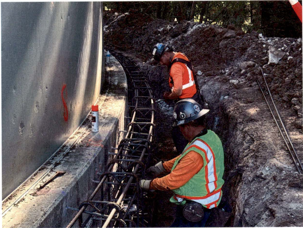
October 29, 2025 – Rebar installation.
