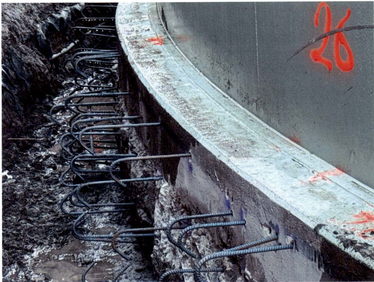
October 17, 2025 – Dowel installation.
