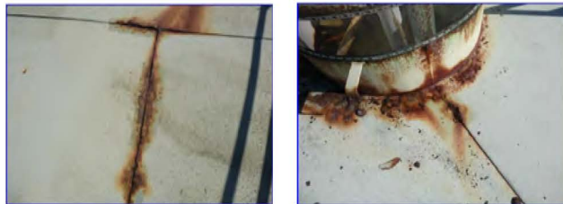
EXTERIOR COATING CORROSION
