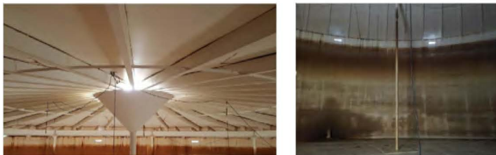
INTERIOR COATING CONDITION
