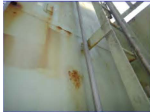
EXTERIOR COATING CORROSION
