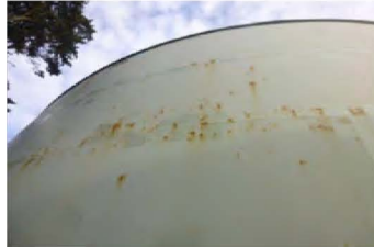
EXTERIOR COATING CORROSION
