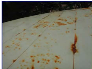
EXTERIOR COATING CORROSION
