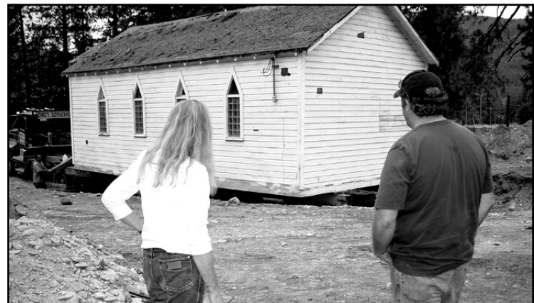
Carol Guthrie and Dave Murray confer as the crew prepares to remove the dollies, leaving the church supported by timbers.
