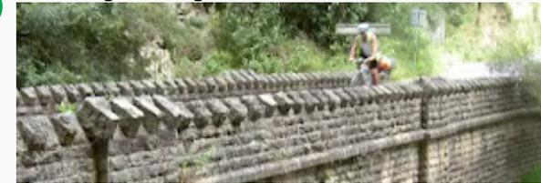
The bridge spanning out from the Grand Arch was designed by Mr Ernest M. De Burgh, and built by the Public Works Department in 1896. The bridge allowed greater access to the caves and was built from locally cut limestone.
