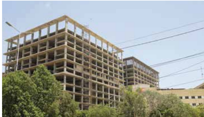
100% GREY STRUCTURE OF HB 1, HB 2 & IUHS COMPLETED
